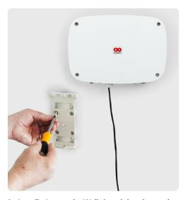
8 Installation on the Wall. Attach bracket to the wall using wall plugs and screws. Than install the enclosure and secure the M4 screw.
